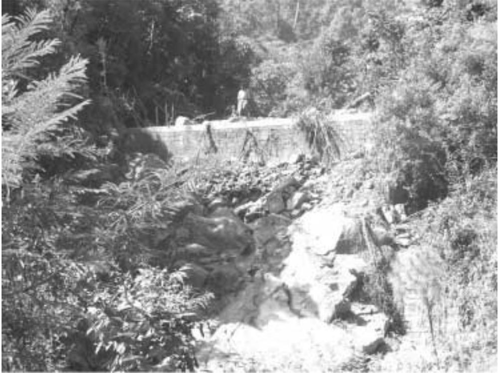
Figure 3. Still intact; upstream view of the structure erected for diverting discharge of the seasonal stream flowing through Amparav to China Gadhera (at (A) in Fig. 2). The structure became silted up and the water overran the structure.
