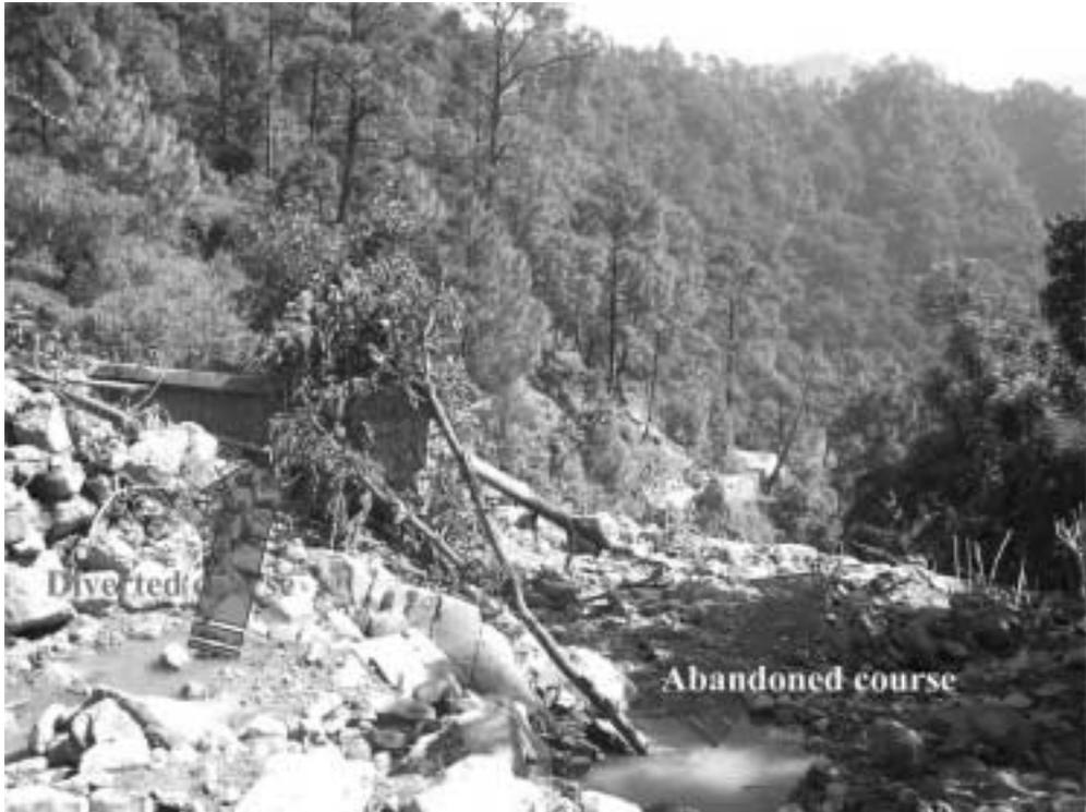
Figure 5. View of the dislodged bridge blocking the course of the diverted stream (at (A) in figure 2).
