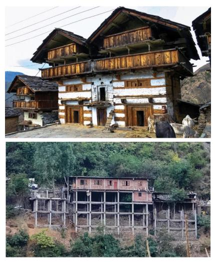
As opposed to traditional structures, a network of illreinforced and unplanned beams and columns that defy the slope of hills of Uttarakhand are in place today. Heavy structures on steep hill slopes are the bane of Devprayag, Karnaprayag, Almora, Rudraprayag and Bhatwari.
