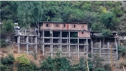
As opposed to traditional structures, a network of ill-reinforced and unplanned beams and columns that defy the slope of hills of Uttarakhand are in place today. Heavy structures on steep hill slopes are the bane of Devprayag, Karnaprayag, Almora, Rudraprayag and Bhatwari.
