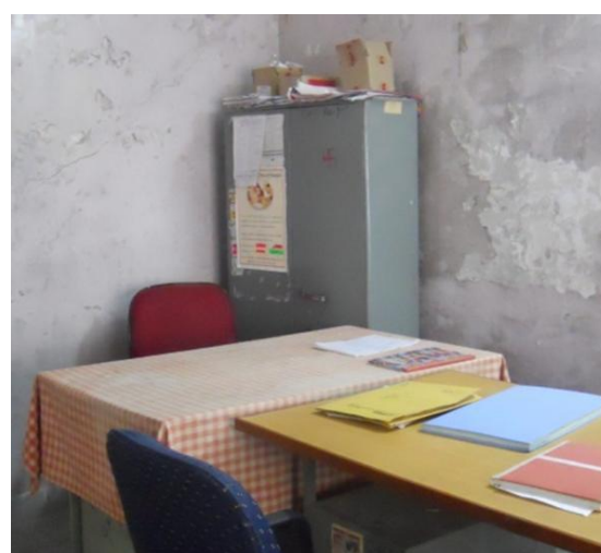
Fig. 44. Cupboard placement in CHC Raipur poses a risk to life safety.
