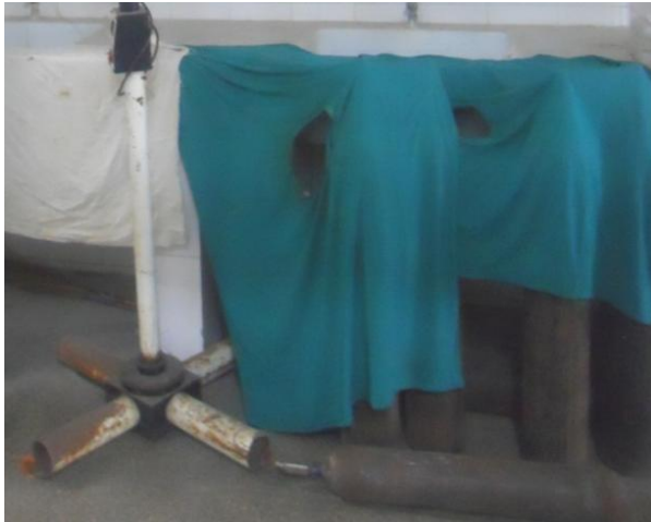
Fig. 58. Unanchored oxygen cylinders outside OT at CHC Vikanagar.
