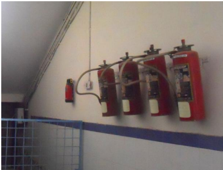
Fig. 60. View of the improperly mounted fire extinguishers at CHC Doiwala.
