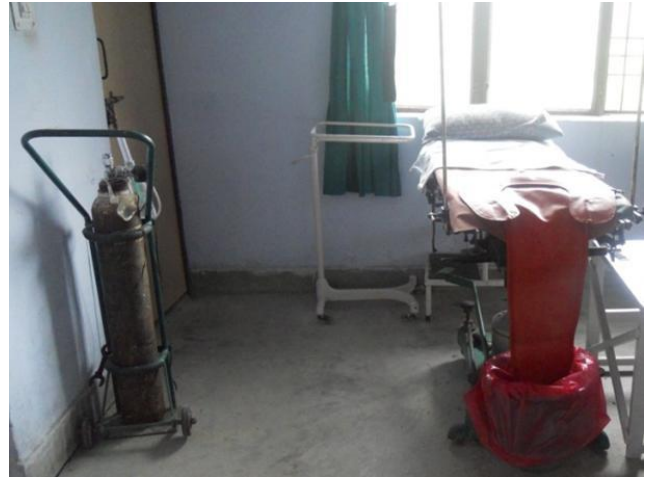
Fig. 59. The Framed oxygen cylinder lacking support from wall at CHC Mussoorie.
