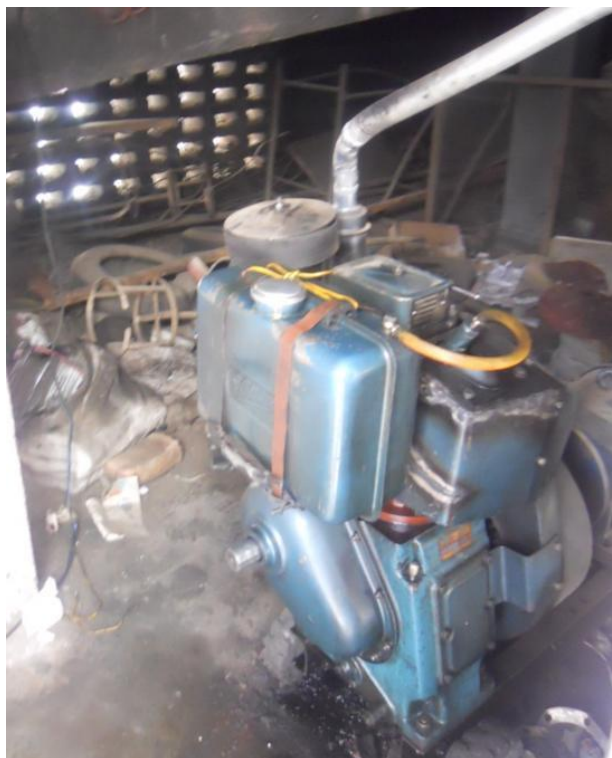
Fig. 49. View of the generator at CHC Vikasnagar. It is required to be anchored to the floor to avoid the danger of its falling down.
