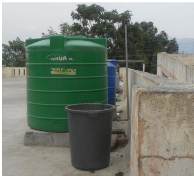
Fig. 55. Unanchored roof water tanks at CHC Vikasnagar.
