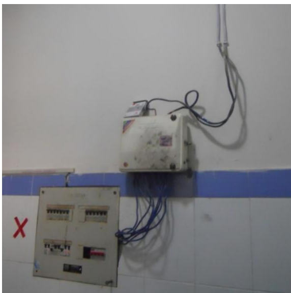
Fig. 54. DB box and the open electric wires at CHC Vikasnagar.
