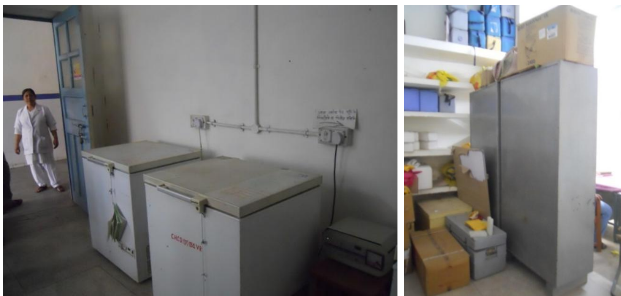
Figs. 35 and 36. View of the freezers at CHC Doiwala that have no anchorage support and the placement of the cupboards in this unit pose life risk to the staff sitting close by.
