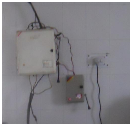
Fig. 53. The electric wires must be properly covered if not it will lead to short circuit , CHC Doiwala.
