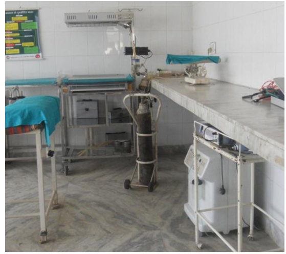
Figs. 23 and 24. View of the labour room at CHC Doiwala. Unanchored oxygenator, baby incubators and oxygen cylinders can be observed in the photograph.
