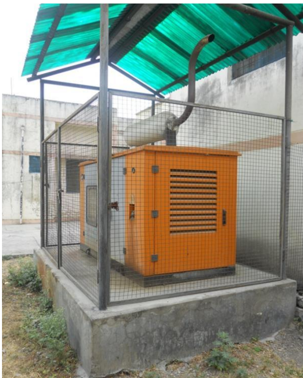
Fig. 48. View of the well fenced and covered generator at CHC Raipur. Additional support at the base would ensure that it does not slip past.
