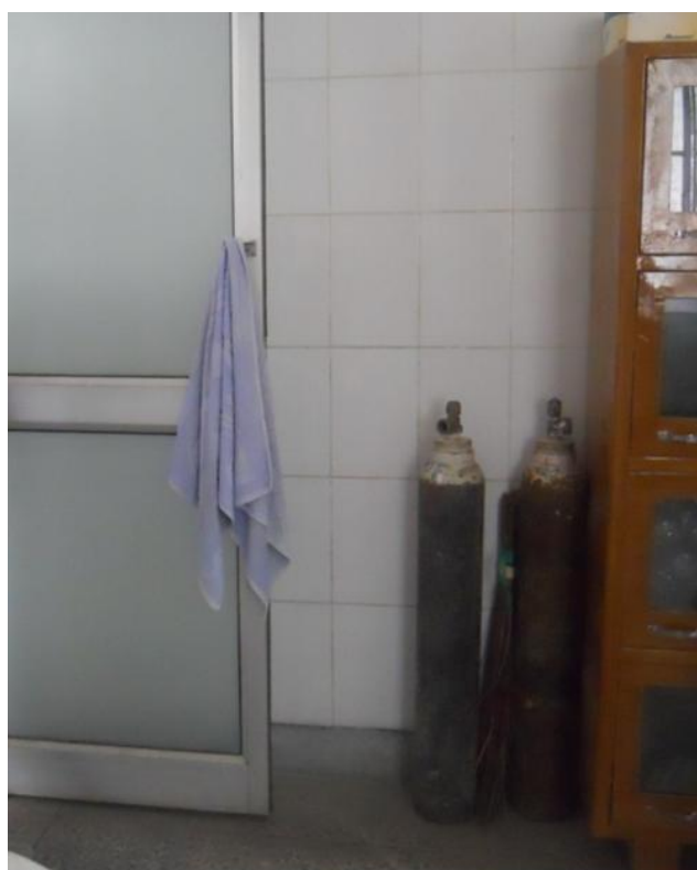
Fig. 56. Cylinders placed without anchorage at CHC Doiwala.
