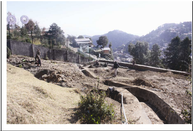
Figure 4 Disposal of excavated debris along the hill slope in Nainital. Obliteration of surface drains by site development works for construction.
