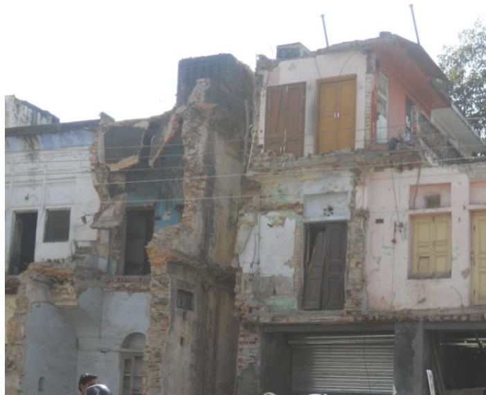
Fig. 13. The new shops being constructed on the ground floor of the partially demolished structure while the upper floors still remain in dilapidated condition.
