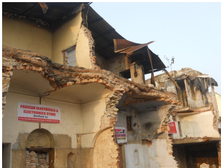
Fig. 10. The damaged segmental arches of the buildings at chakrata road.
