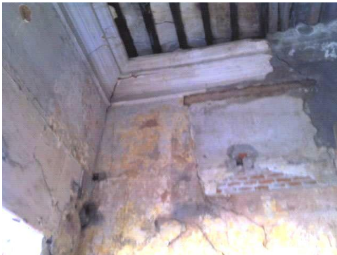
Fig. 8. The cracks developed on inner walls of the building.
