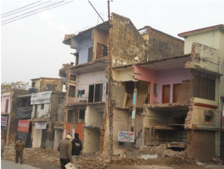
Figs. 14 and 15. The load bearing masonry construction with RB roofs to the north of the Chakrata Road.
