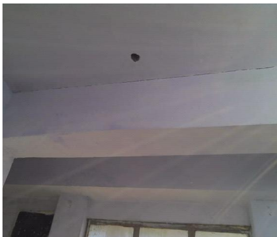
Figs. 25 and 26. Cracks developed along beam and arches because of lack of systematic approach followed in demolition.
