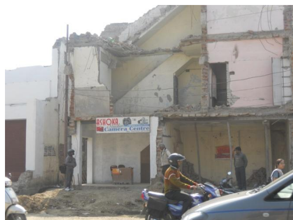
Fig. 23. Ground floor construction with weak upper storeys can lead to a disastrous situation.
