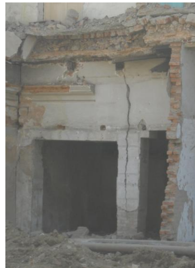
Fig. 9. Highly vulnerable structures with multiple weaknesses must be fully demolished to avoid the risk.
