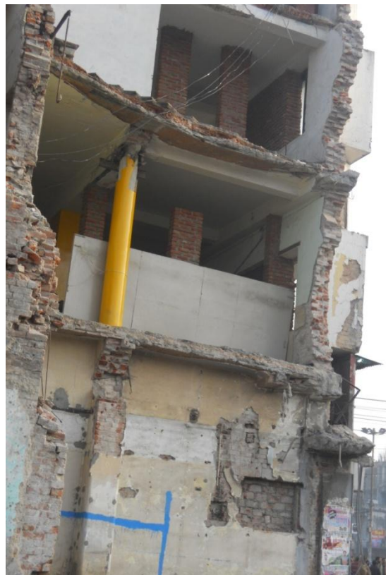
Fig. 29. No proper hierarchy of columns being followed in construction which will lead to structural instability.
