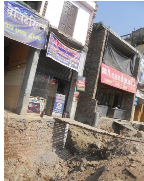
Figs. 20 and 21. Drainage work in progress along with the poorly placed wooded planks to ensure customer access.
