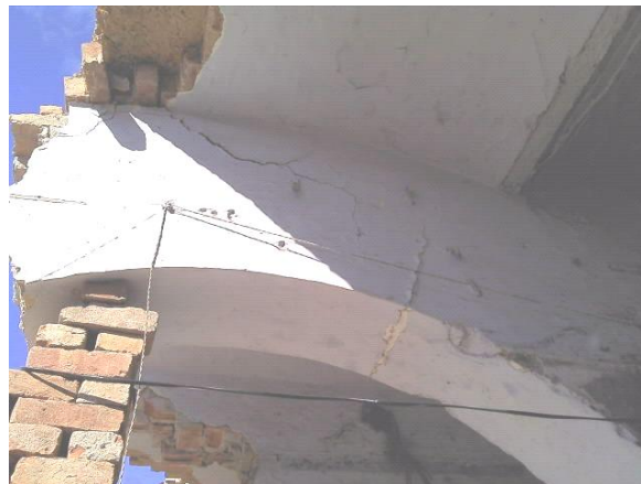
Fig. 16. The cracks developed in the partially demolished building enhancing its structural vulnerability.
