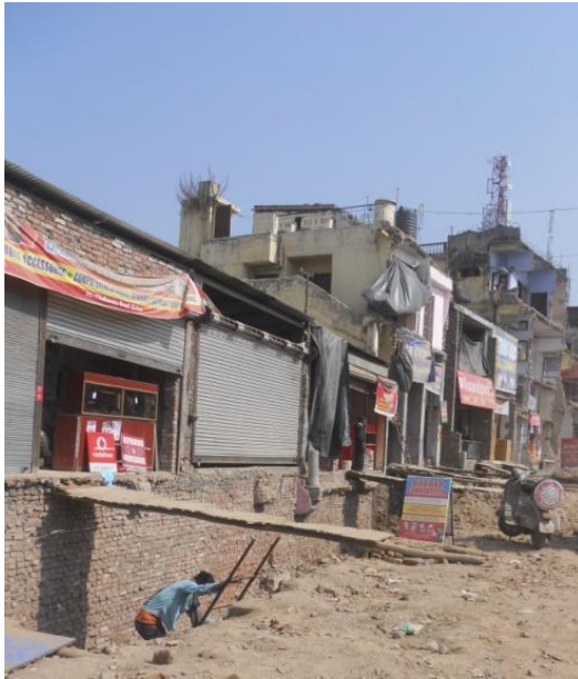
Figs. 20 and 21. Drainage work in progress along with the poorly placed wooded planks to ensure customer access.
