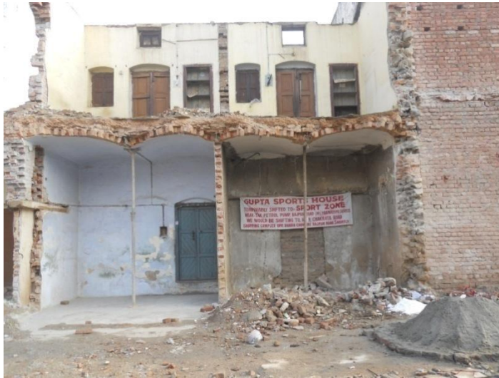
Fig. 17. The damaged arches and the load of arches being supported by being planks.
