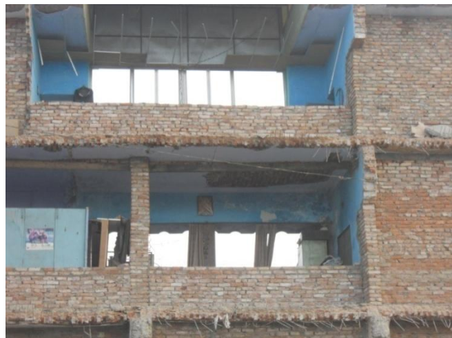
Figs. 18 and 19. The new construction practice at the site; irregular / tilted columns being constructed.
