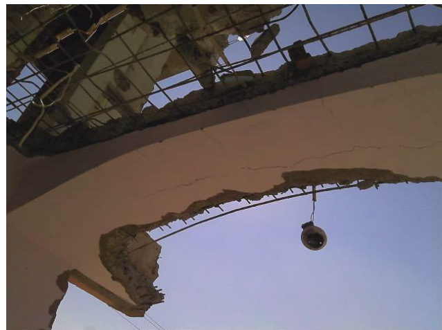
Figs. 25 and 26. Cracks developed along beam and arches because of lack of systematic approach followed in demolition.
