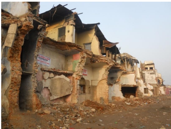
Fig. 6. The old structures on the southern side of the Chakrata Road made mostly of Lahori bricks.
