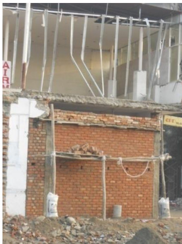
Figs. 18 and 19. The new construction practice at the site; irregular / tilted columns being constructed.
