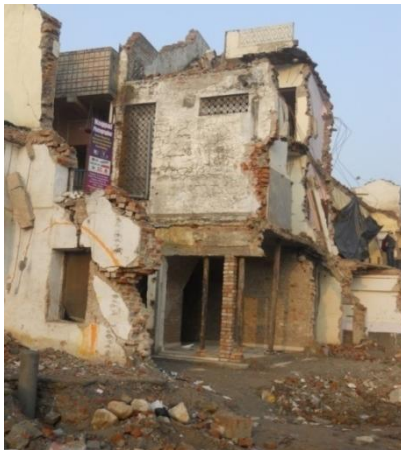
Fig. 11. The vertical columns being erected to support the hanging roof.
