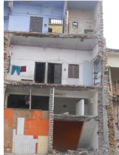
Figs. 14 and 15. The load bearing masonry construction with RB roofs to the north of the Chakrata Road.
