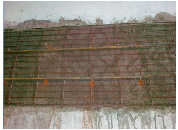
Fig. 35: Figure showing fitting of wire mesh and reinforcement bars.
