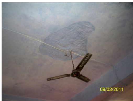
Fig. 12: View of oneycombing in the roof of the structure.
