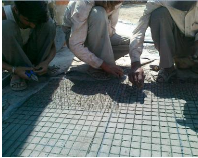
Fig. 44: Binding wire being inserted into the spacers.
