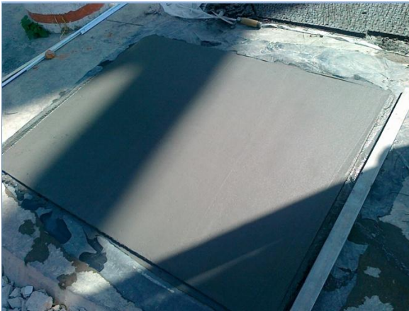
Fig. 42: Figure showing the base from which spacer is made; the base is 15 mm thick.
