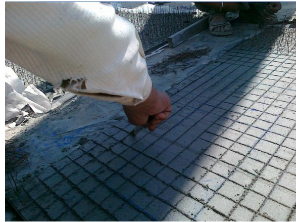
Fig. 43: Figure showing cutting of spacers (2" x 2").
