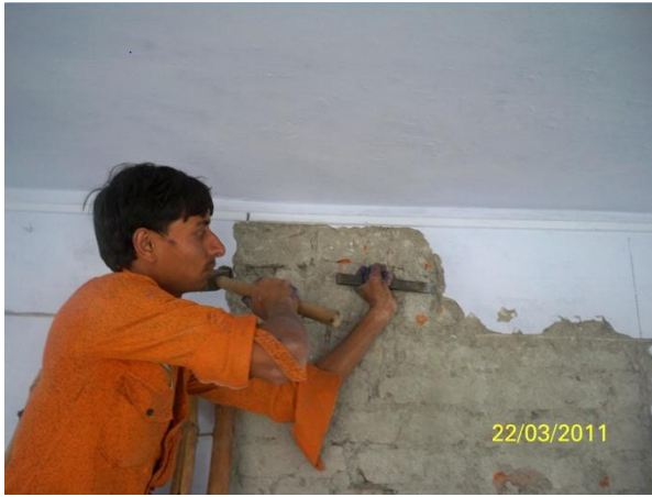
Fig. 24: Mason using chisel and hammer to chip off the plaster.
