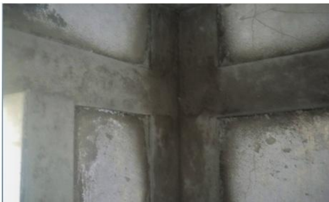
Fig. 40: The final finished look of the wall after plastering.
