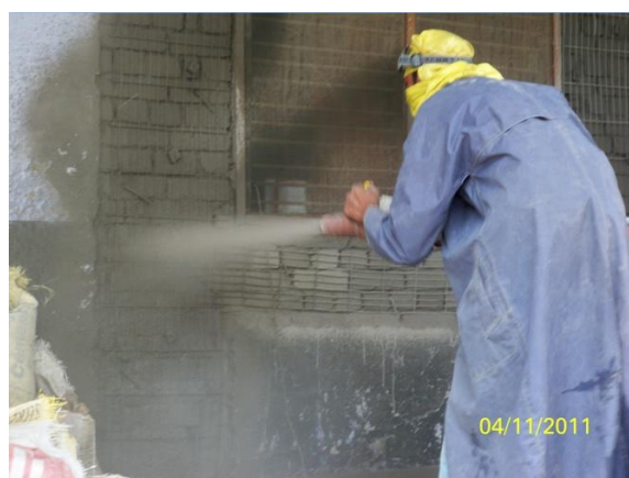
Fig. 51: Micro-concrete coming out at high velocity from the nozzle.
