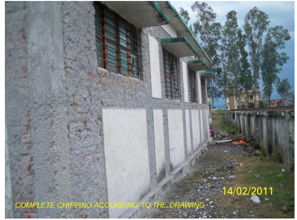
Fig. 25: Figure showing complete chipping according to the drawing.
