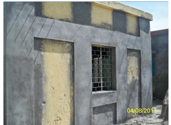
Fig. 41: The final finished look of the wall after plastering.
