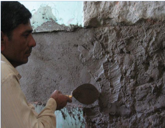
Fig. 32: Mason applying first layer of cement mortar.
