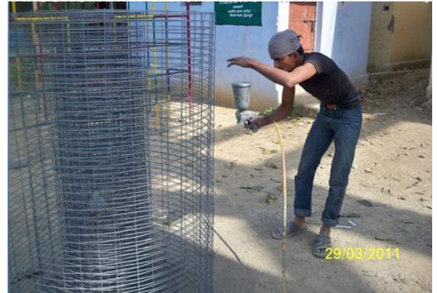
Fig. 29: Figure 4(a): Mason applying epoxy primer using spray.
