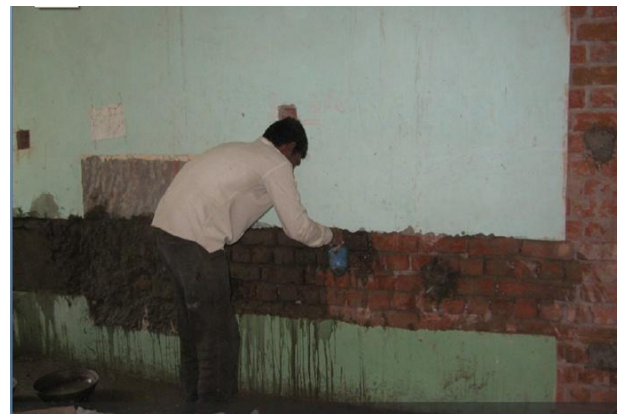
Fig. 31: Mason applying cement slurry on wall.
