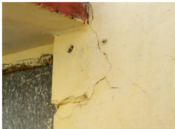
Fig. 15: Shear / diagonal crack observed in the school building at Dobhalwala.
