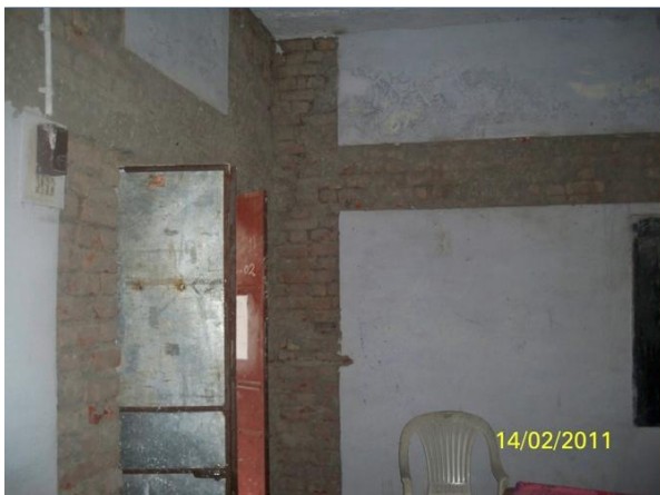
Fig. 26: Figure showing complete chipping of plaster inside the room.
