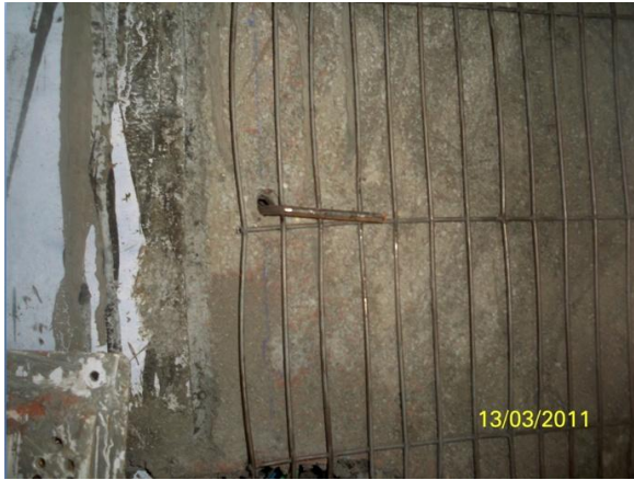
Fig. 34: Wire mesh being held in position using 6 mm steel bars.
