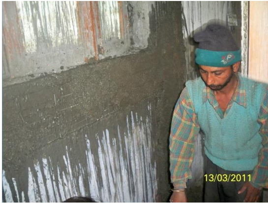
Fig. 28: Mason applying second layer of micro-concrete.
