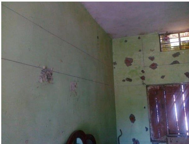
Fig. 22: Markings being done using blue colour and thread.
