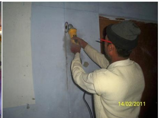
Fig. 23: Mason using stone cutting machine to chip off at markings.
