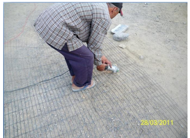
Fig. 27: Mason using rotating cutter to cut wire mesh.
