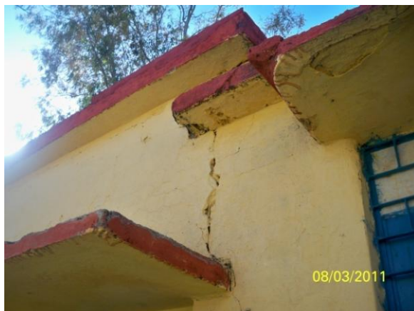
Fig. 14: Joint crack observed in the school building at Dobhalwala.
