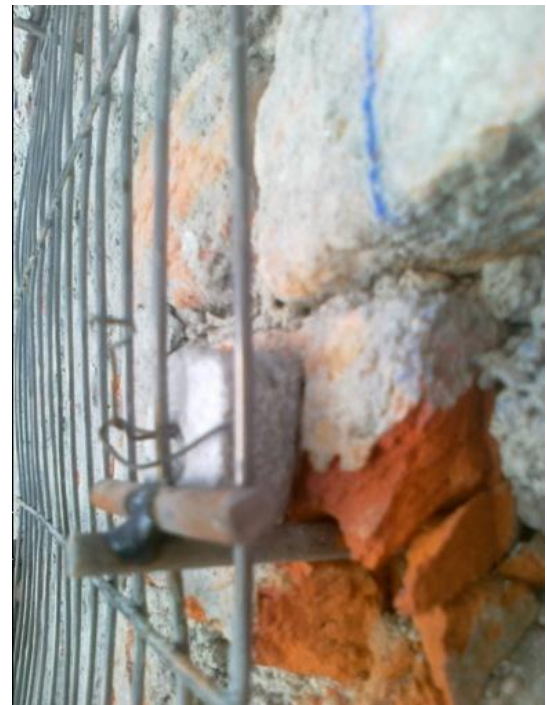
Fig. 48: A spacer tied between the wall and the mesh.
