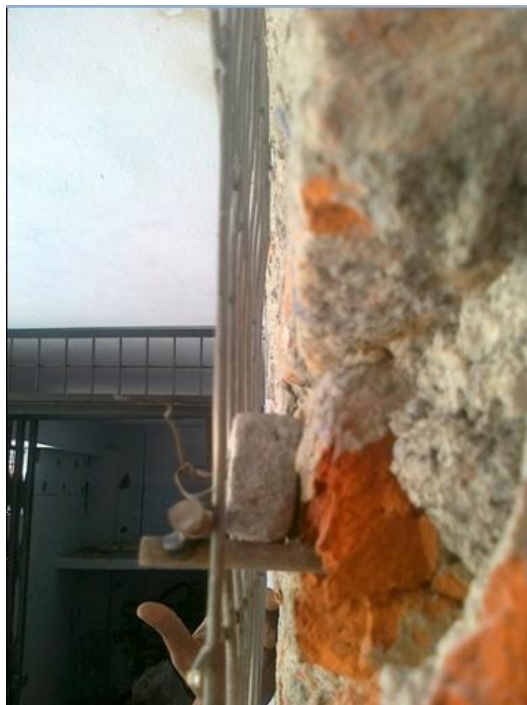
Fig. 47: A spacer tied between the wall and the mesh.
