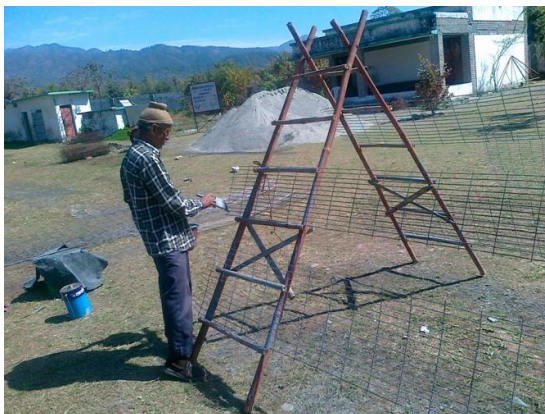
Fig. 30: Mason applying epoxy primer using paint brush.
