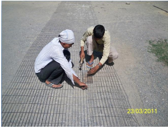
Fig. 28: Masons using chisel and hammer to cut wire mesh.
