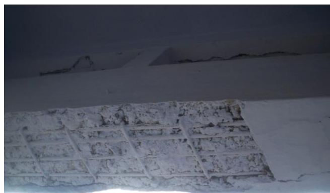
Fig. 13: Exposed steel reinforcement of the roof.
