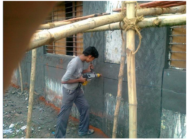
Fig. 33: Mason drilling holes into the wall.
