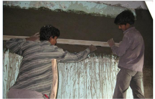
Fig. 29: Mason applying third and the final layer of plaster.
