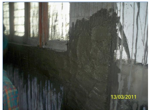
Fig. 37: View of the second layer of micro-concreting.
