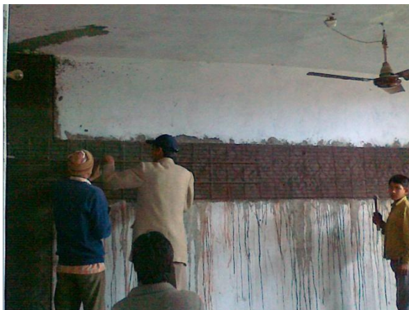
Fig. 36: Masons fitting the wire mesh and reinforcement bars.
