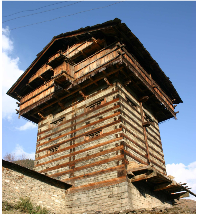
Fig.10: The vertical wooden beam on the side walls is considered to be a seismic safety related provision.
