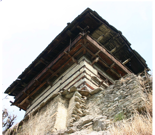
Fig. 7: Raised platform erected over in situ rocks to support the multi-storied structure.
