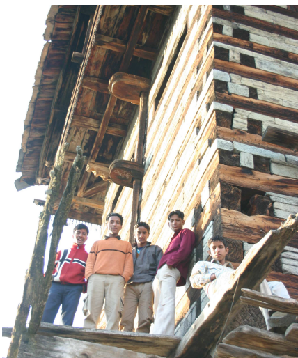
Fig.9: Wood – stone architecture of the walls of the traditional multi-storied structures.
