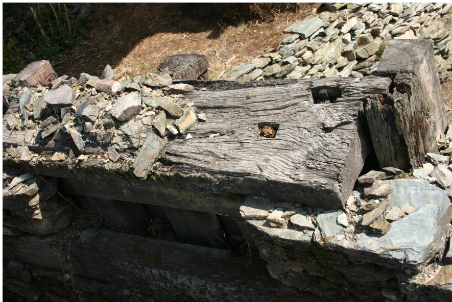
Fig.11: Housed and nailed joints used for fixing the wooden components of Koti Banal architecture.
