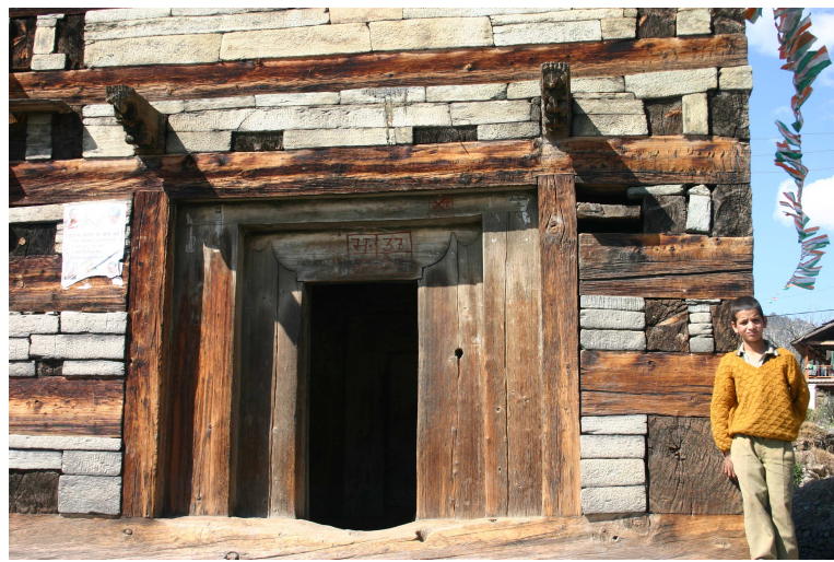
Fig.9: Wood – stone architecture of the walls of the traditional multi-storied structures.
